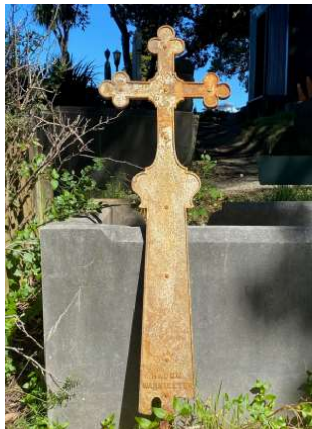
The broken Prichard cross (above) has been repaired very recently, and will be reinstated soon in the upper Cemetery.
