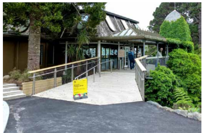
Before and after photos of the Treehouse ramp refurbishment.
